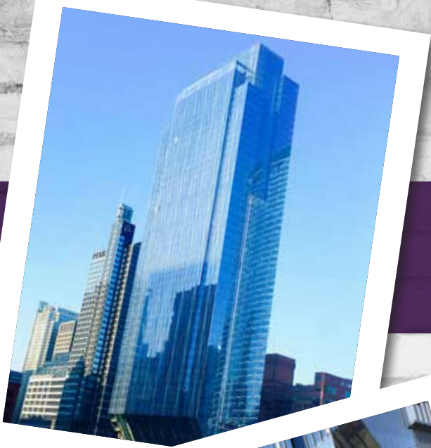
150 NORTH RIVERSIDE PLAZA 1.3M RSF
