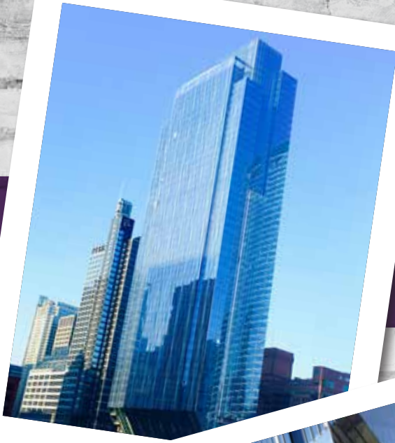
150 NORTH RIVERSIDE PLAZA 1.3M RSF
